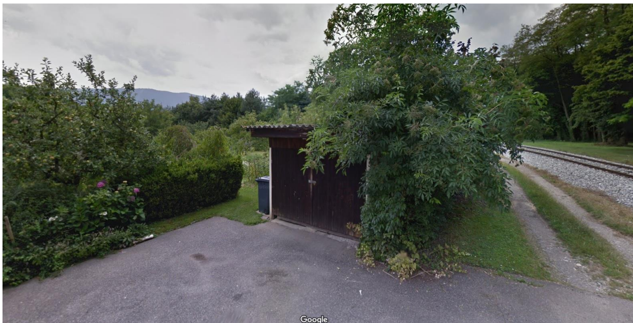
Slika 8: Pogled na obstoječe stanje proti jugu, ob železnici, vir: https://www.google.com/maps
